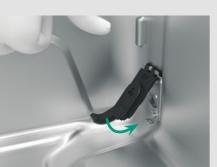
I Place condensate outlet back in position (snaps into place).
